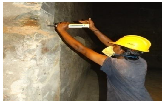
Figure 1: Rebound Hammer in Progress
