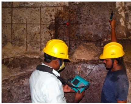
Figure 7: Half-cell Potential Test in Progress
