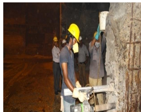
Figure 3: Core Extraction in Progress
