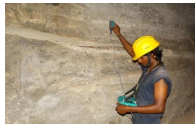
Figure 5: Cover Meter Test in Progress
